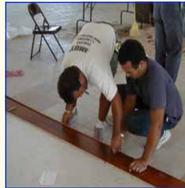
BUILDING THE “NEW” OUR LADY OF MT. CARMEL
